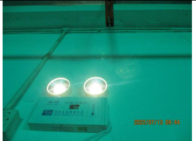
Emergency light test
